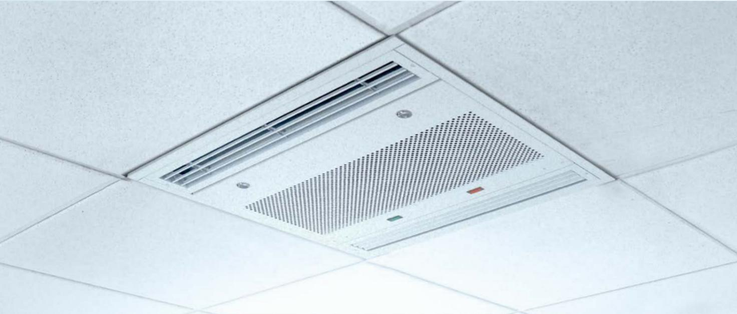
Our Ceiling Cassette is a versatile UV air purifier which fits seamlessly into the environment. Concealed above the ceiling, the Cassette quietly removes harmful virus and bacteria, delivering clean, purified air into the space.
